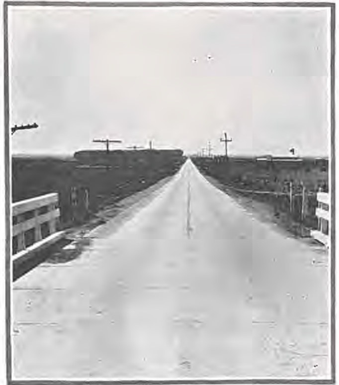
A section of the Federal Aid concrete pavement south of Sterling, in Logan county. This road serves a rich irrigated agricultural section, and also carries large tourist traffic from the east. The paving between Sterling and Fort Mogan will be completed this summer, a distance of about thirty miles.
