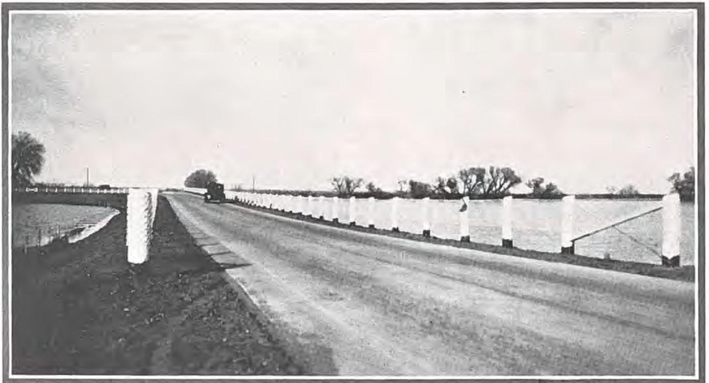
Showing Newly Completed Concrete Pavement Crossing Lake, North of Lafayette
