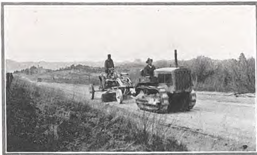
One of the new state maintenance tractor-grader outfits smoothing out the "wrinkles" on road north of Monument in El Paso county.
