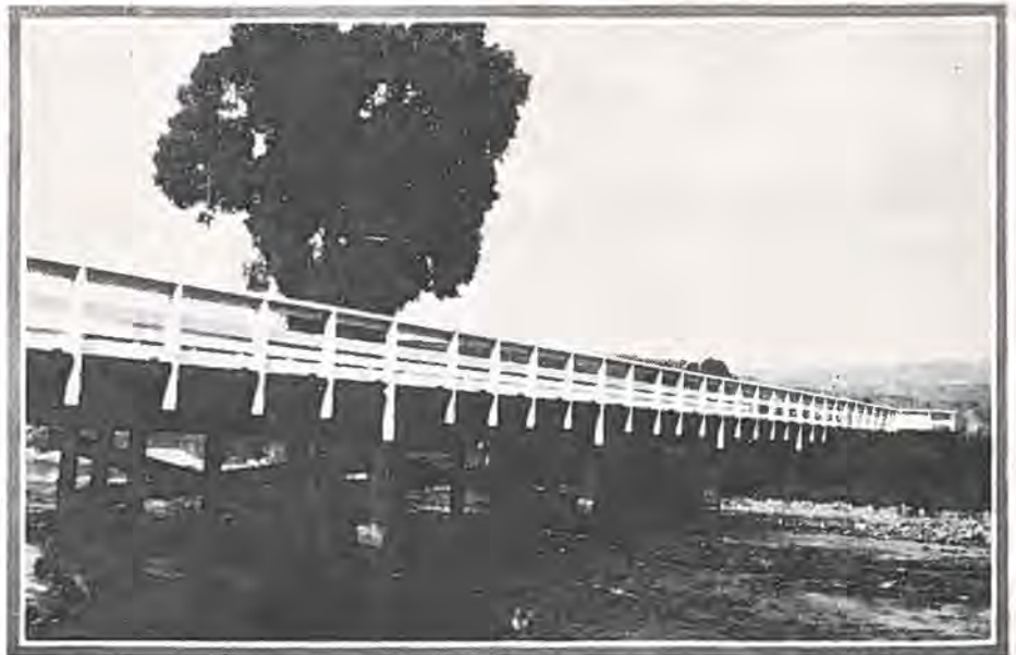
Treated timber bridge near Milner, one of many such structures being constructed by State Highway Department.
