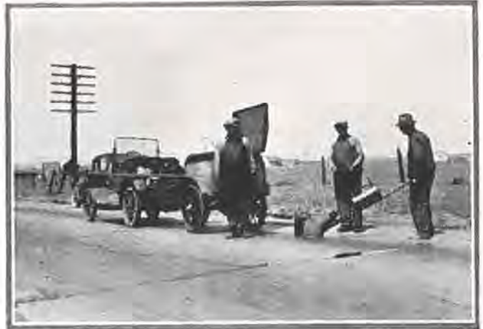
State force making repairs on Denver-Golden pavement—now in splendid condition.
