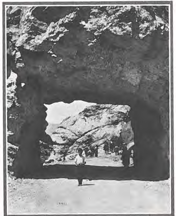
A short tunnel on the Canon City-Salida highway, or Rainbow Route, in Fremont County. Photos by H. P. Wilson.
