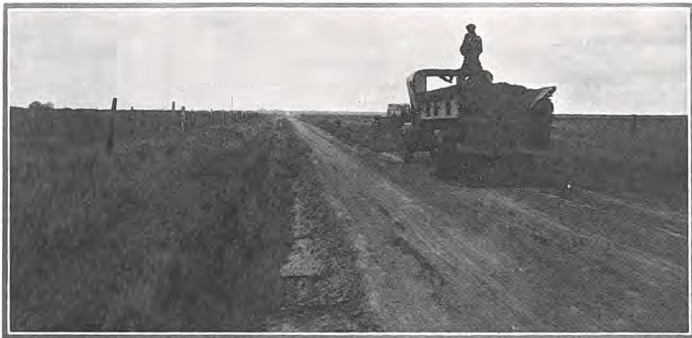
Showing a county truck spreading gravel on State Aid Road No. 51, north of Wray, in Yuma county. This road forms a part of Yuma county's splendid gravel road system.
