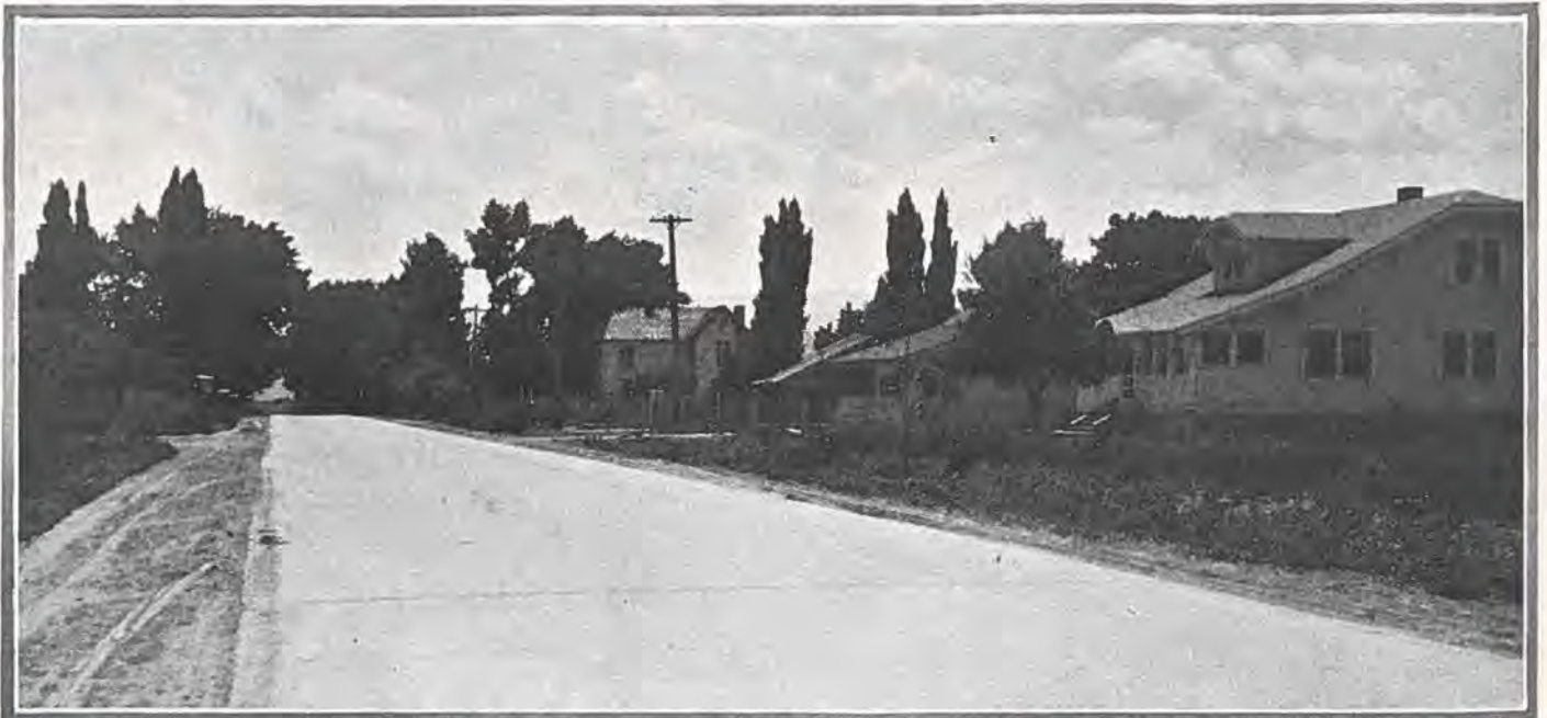
Showing concrete road between Grand Junction and Palisade, in Mesa County, serving a rich farming community.
