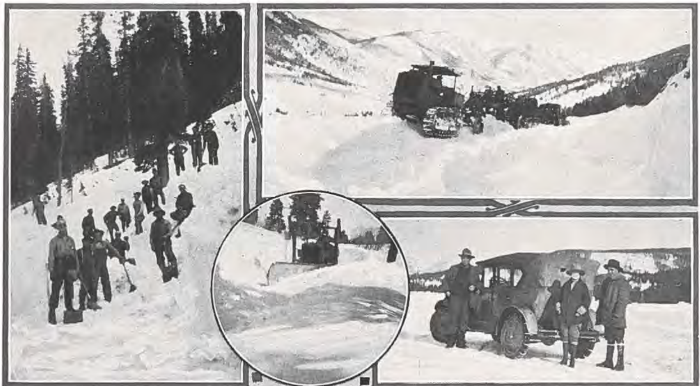
Snow removal scenes in Colorado during the month of June. Left—Shovel crew on west slope of Berthoud Pass. Upper right—Tractor-grader outfit clearing road on Tennessee Pass. Circle—Caterpillar with Killefer power control plow opening road near Electra Lake, above Durango. Lower left—Midwinter tourist party on summit of Tennessee Pass.
