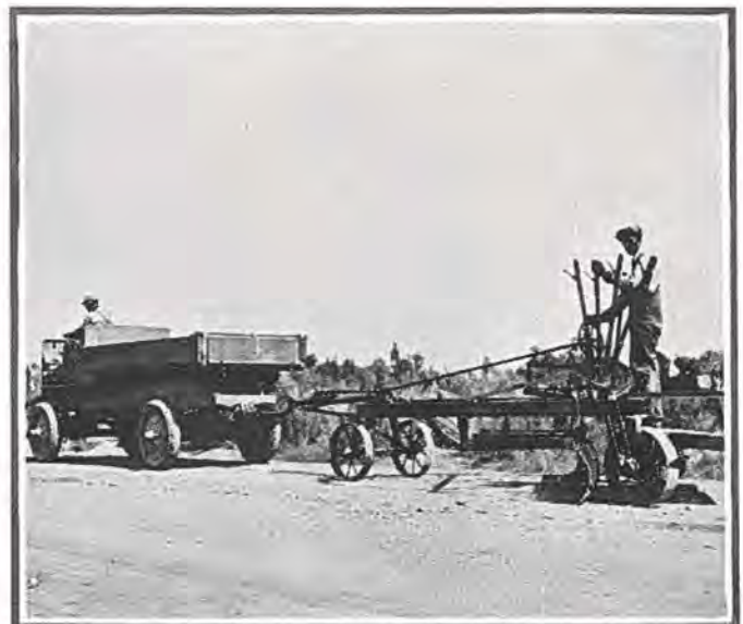
One of Montrose County's maintenance crews working on State Road No. 6
