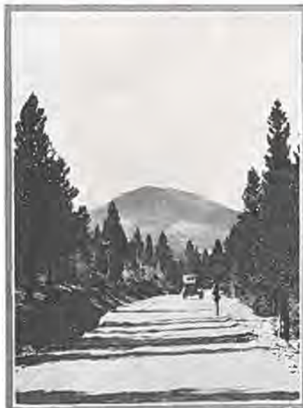
Showing section of Cumbres Pass highway recently completed by U. S. Forest Service.
