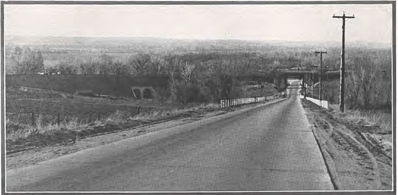
Concrete pavement near Wolhurst on State Road No. 1, showing how sixteen grade crossings are being eliminated between Denver and Colorado Springs by the State Highway Department.
