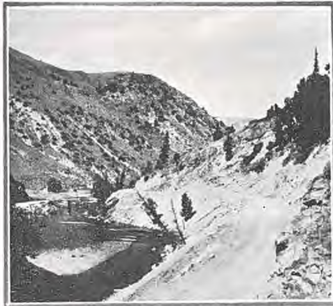
A view of Byers canyon, Federal Aid project recently opened to traffic. Note heavy rock excavation. Colorado river on left.
