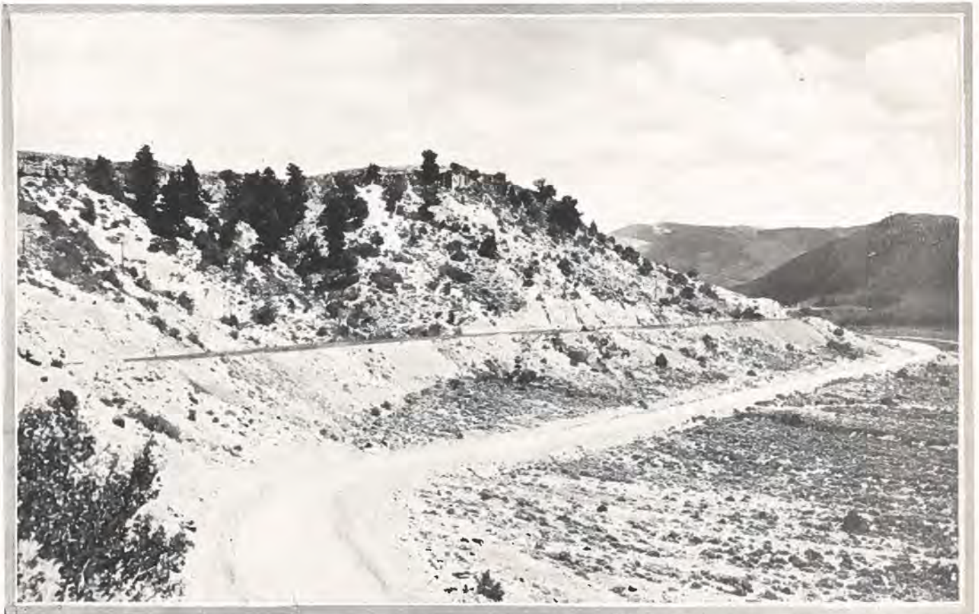
Where the motorist may race a train, and without a grade crossing. The scene is in Grand County, showing the new state highway paralleling the Moffat railroad, shown along the side of the mountain. This is a graveled road between Byers Canon and Parshall.
