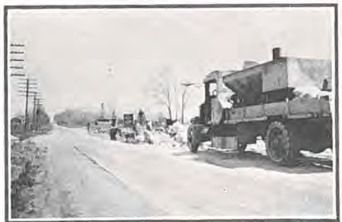
State Maintenance Crew Repairing Golden Pavement, Two Miles West of Denver
