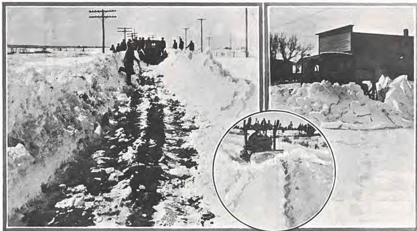
Snow removal scenes in Eastern Colorado. Left—Showing crew at work in Sedgwick county. Right—Bucking snow in the town of Sedgwick. Circle—Clearing road west of Durango in La Plata county.
