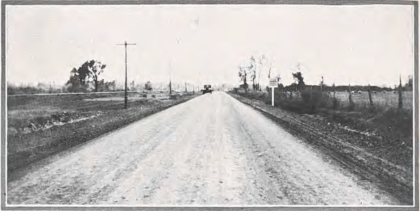
Showing a stretch of the newly completed oil processed highway near Romero in Conejos County.
