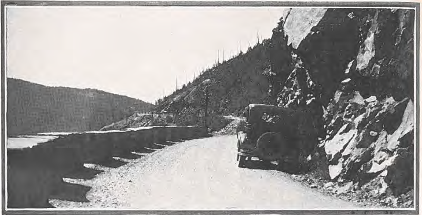
A stretch of protected road on Colorado's Million Dollar Highway, located on Cascade Divide in San Juan County. From the edge of the protection to the bed of the canon it is 800 feet. Photo by B. B. Allen.
