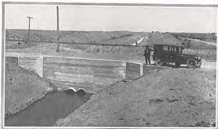
Section of State Road No. 1, south of Pueblo, showing unusual culvert installation.
