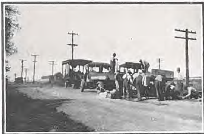
Showing Arapahoe County Crew Making Repairs on Denver-Littleton Pavement
