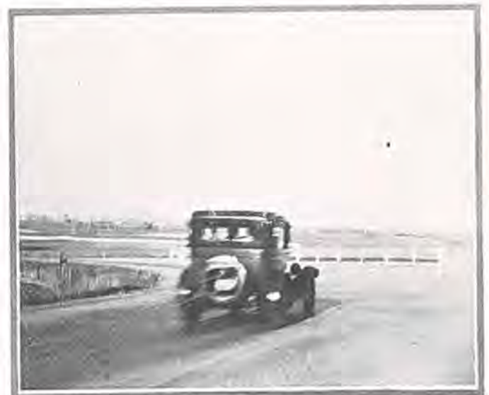
Showing new guard fence at "Dead Man's Curve" on Denver-Morrison pavement. No accidents have occurred at this turn since installation of fence.
