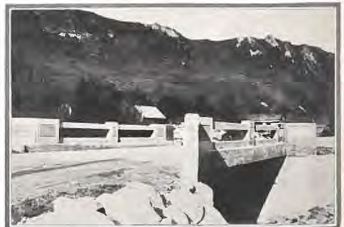
No slowing down for bridges on completed state highway projects. This bridge at Aspen is typical of construction of such structures on all Colorado state roads.
