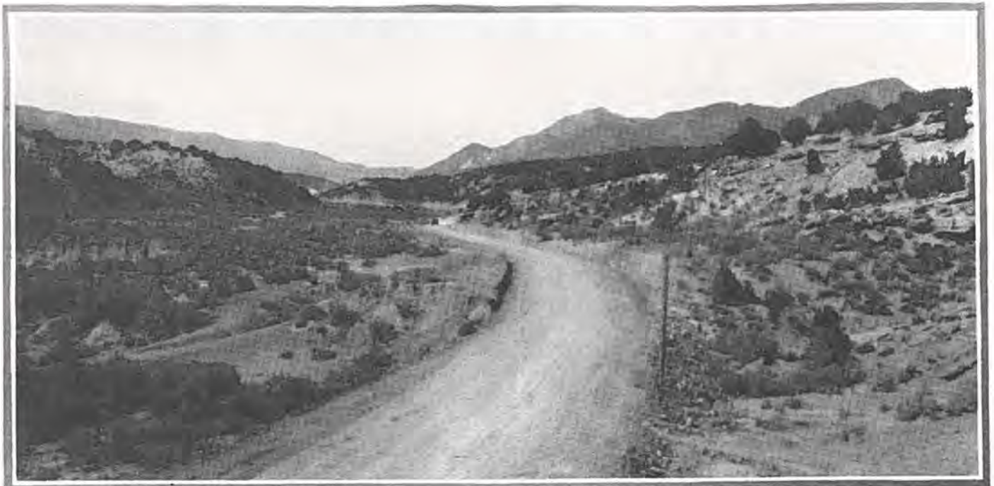
Showing a fine stretch of gravel surfaced highway near Grand Valley in Garfield county, recently finished with Federal Aid funds. This road is a part of "U. S. Highway 40—south." Photo by H. L. Jenness.
