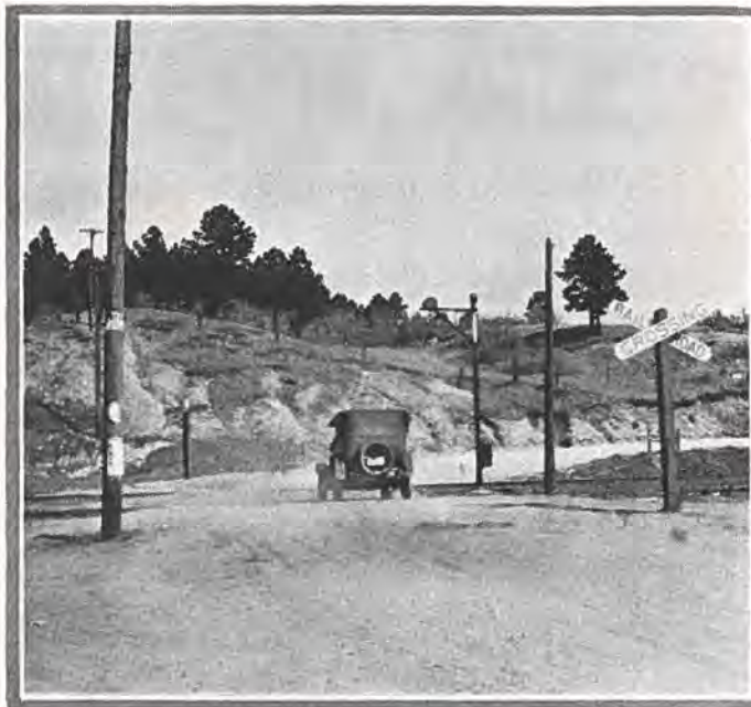
One of the six railroad underpass crossings constructed under the supervision of the state on the Denver and Colorado Springs paved highway. Several persons were killed at the crossing which this underpass eliminates. During the past seven years more than sixty dangerous railroad crossings have been eliminated in Colorado by the construction of underpasses such as that pictured above, or through realignment of the roads.
