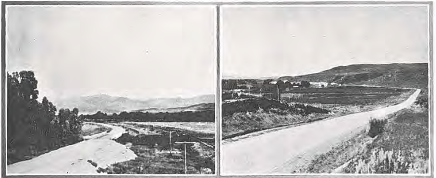
Two views of the Victory Highway. On left, a picture of new Federal Aid highway west of Milner; on the right, another completed Federal Aid project west of Craig. Photos by H. L. Jenness, division engineer.
