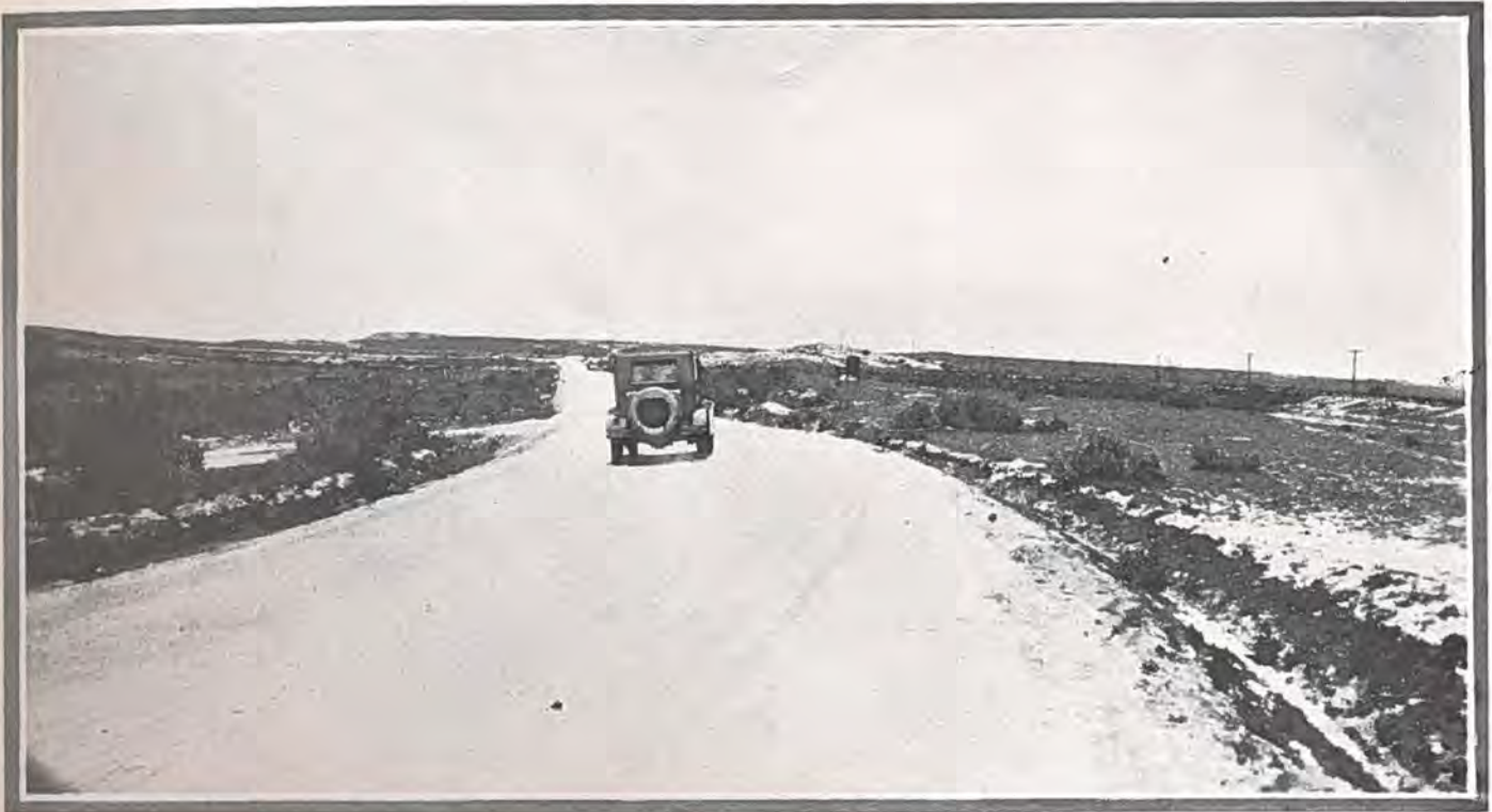
An Improved Stretch of Gravel Surfaced State Highway West of Pueblo
