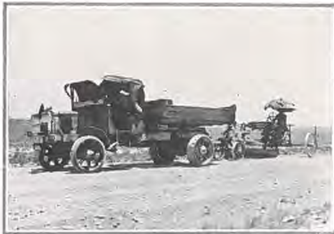
Keeping the road smooth between Pueblo and Florence for the heavy summer traffic.
