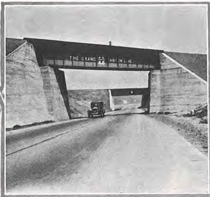
One of the six railroad underpass crossings constructed under the supervision of the state on the Denver and Colorado Springs paved highway. Several persons were killed at the crossing which this underpass eliminates. During the past seven years more than sixty dangerous railroad crossings have been eliminated in Colorado by the construction of underpasses such as that pictured above, or through realignment of the roads.
