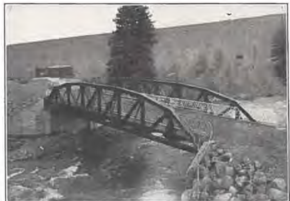
100 ft. Riveted Low Truss Span, Dillon, Colo.
