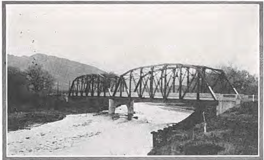
State highway bridge south of Colorado Springs, over the Fountain river. A five-mile stretch of concrete pavement is being constructed by the Highway Department, connecting with this bridge on the south.
