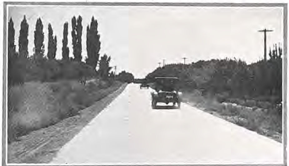
Concrete paved road through fruit-growing section near Palisade, in Mesa county, constructed with Federal aid.
