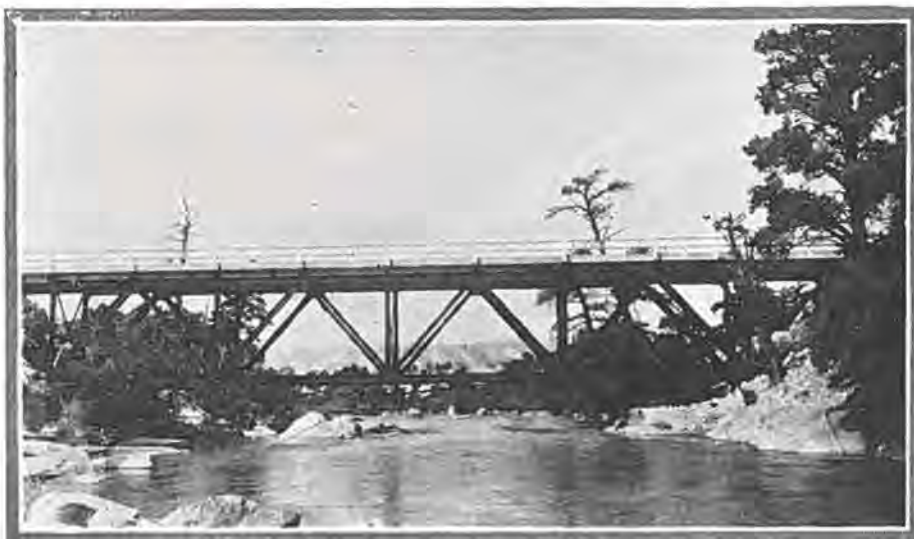
Steel highway bridge which spans the Arkansas river near Salida, in Chaffee county, constructed with Federal Aid funds.
