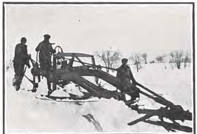
One of Adams County's Maintenance Crews Removing Snow East of Brighton
