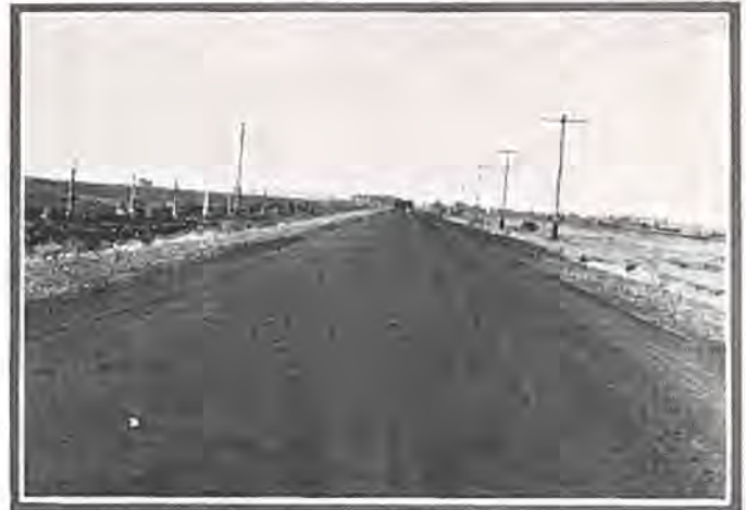
A stretch of oil processed road northwest of Alamosa, recently completed under state supervision. Photo by J. W. Walsh.
